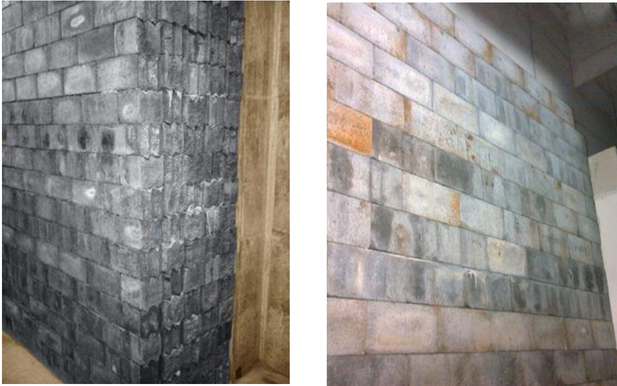
Figure 21 Interlocking HD Block ( left ), Straight Grouted HD Block ( right )
