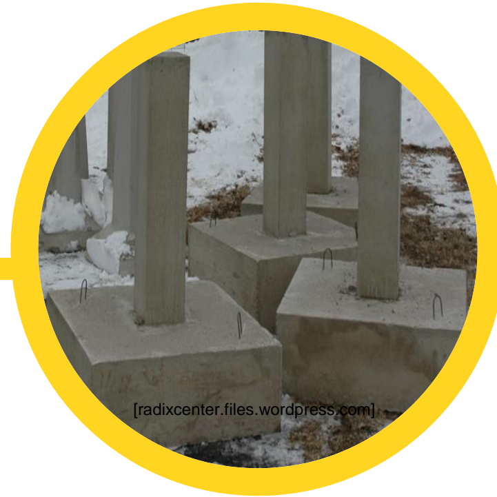
Analysis II | Precast Footings Not Recommended
