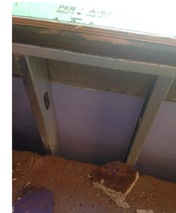
Exterior Wall Assembly |
