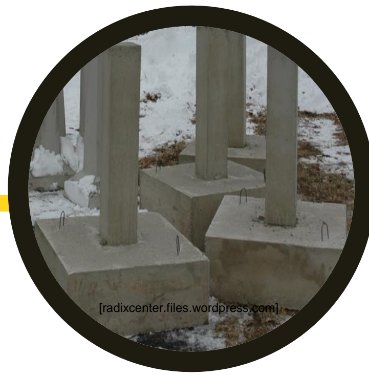
Analysis II | Precast Footings ✗ Not Recommended
